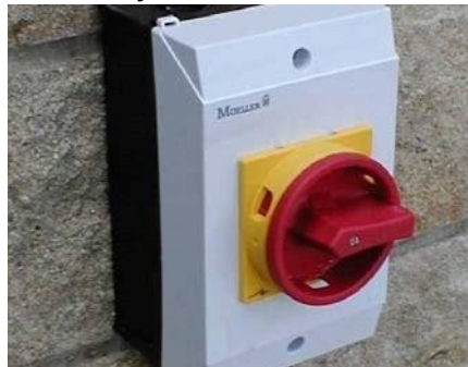
Rotary Isolation Switch
