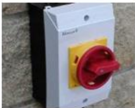
Rotary Isolation Switch
